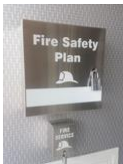
Recommended Fire Safety Plan Box & Key Box
